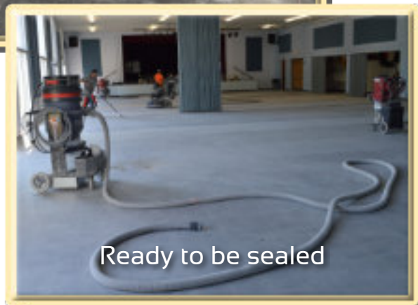
Prepping the concrete
